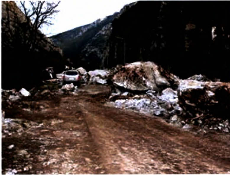
Photo 1 The Greek National Road (PATHE) after the rock fall
