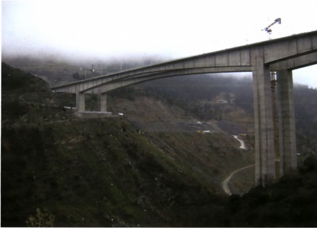
Figure 5.20: General view of Metsovo ravine bridge (November 2008)
