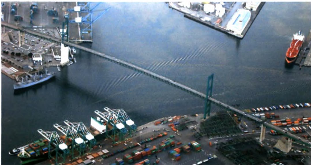
Figure 17: View of Vincent Thomas Bridge
