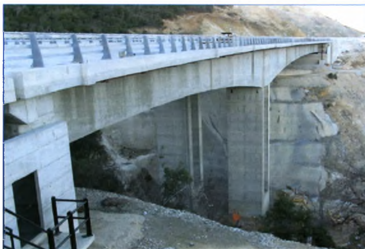
Figure 9: View of Polymylos bridge
