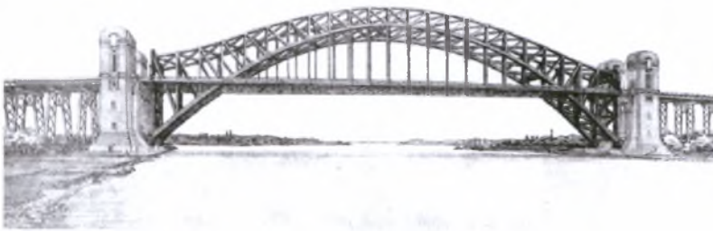
Span 1,000 Feet, Width 91 Feet, Rise of Arch 220 Feet, Maximum Depth of Truss 140 Feet. THE LARGEST ARCH BRIDGE IN THE WORLD CROSSING EAST RIVER AT HELL GATE.
