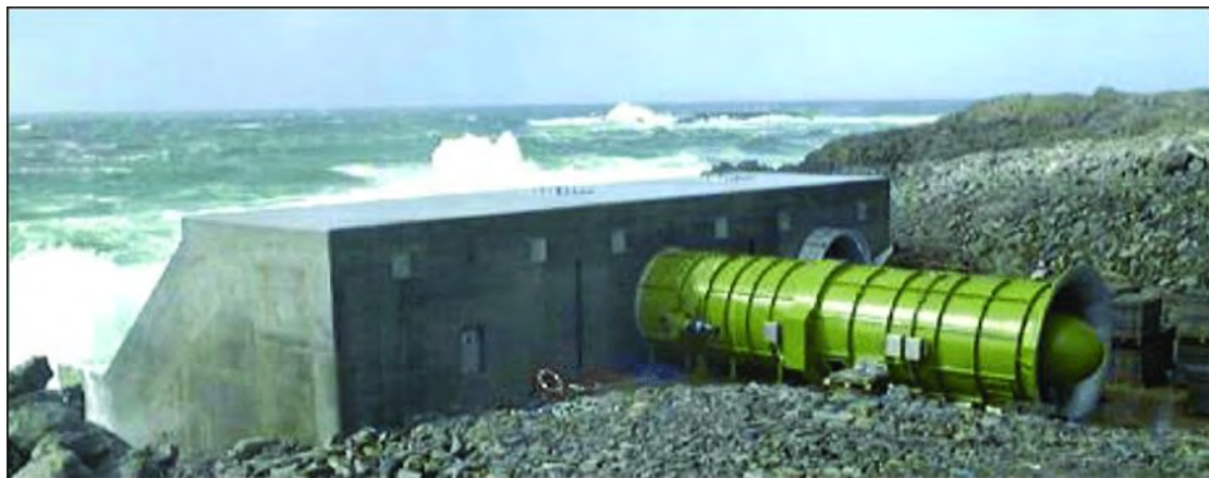
Εικόνα 1-2: LIMPET OWC plant, rated 500 kW, installed in 2000 on the island of Islay
