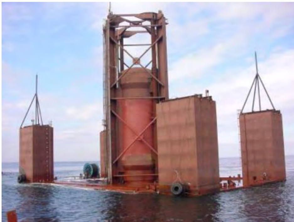
Εικόνα 1-4: AWS installed off Orkney in 2007 by AWS Ocean Energy with eventual plans to create 250kW Πηγή: https://teamwork.nl/front-page/twt/portfolio/aws-2/
