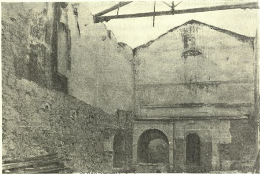
Εἰκ. 1. Ἀποψὶς τοῦ ἐσωτερικοῦ τοῦ ναοῦ ἀπὸ Α μετὰ τὴν μερικὴν ἀφαίρεσιν τῶν κονιαμάτων.
