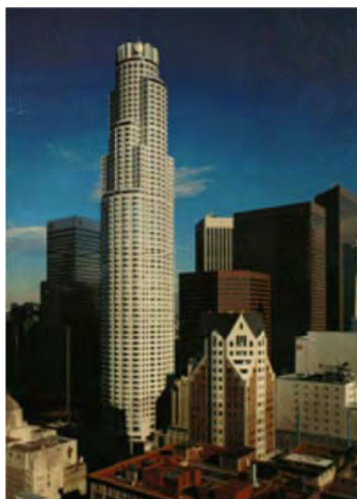
At 1,018 feet, First Interstate World Center, a Maguire Thomas Partners. Project is the worlds' tallest building in a seismic zone 4 or equivalent. Structural Engineering by CBM Engineers, Inc., Houston, Texas.
