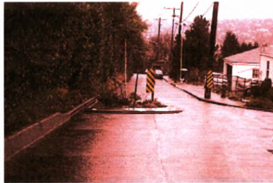
Φωτ. Realigned Intersection
