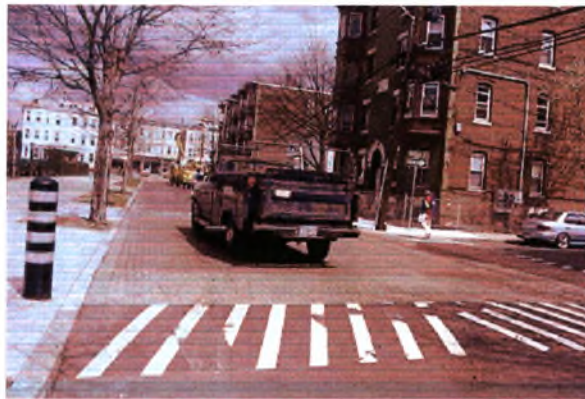
Φωτ. Raised Intersection
