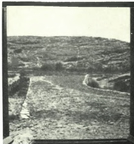
Kea. Ayia Irini : a. Rooms XIII and XV. Repairs and buttresses, marked with whitewash, b. Guardhouse and workrooms, from the South, c. View from east window of guardhouse towards the new road built by the excavators in 1963 - 1964. This is the public road from Vourkari and Korissia
