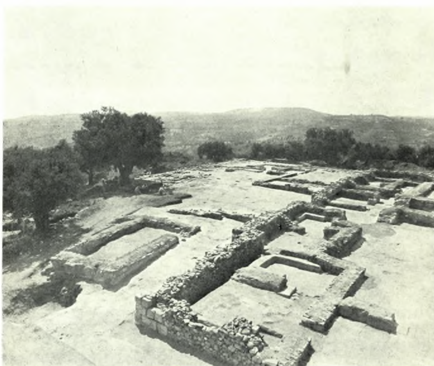
Pylos: a. Southeastern part of the Southwest Wing ( from West ), b. Southwestern Wing of Palace ( from East )
