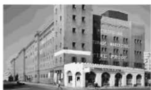
Metropolitan Warehouse Renovation
