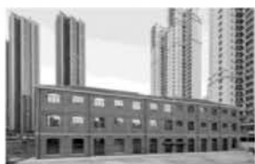
Xintai Warehouse Renovation
