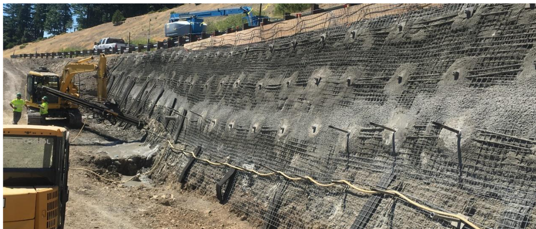
Εικόνα 33: Τεχνική, soil nailing stabilization. https://www.geostabilization.com/wp-content/uploads/2024/02/AL-Soil-Nail-Wall-Banner-scaled.jpg
