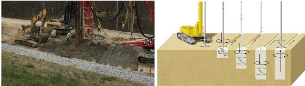
Εικόνα 32: Deep Mixing (Baθiά Enίσxuxh). https://ars.els-cdn.com/content/image/3-s2.0-B978012408076800011X-f11-10-9780124080768.jpg https://www.researchgate.net/publication/337195301/figure/fig2/AS:824424089542656@1573569428349/Deep-soil-mixing-for-shear-wall-installation-at-toe-of-ash-pond-embankment.jpg
