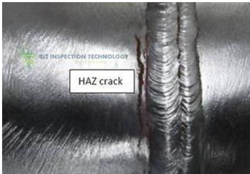
Εικόνα 16:Cracking in Heat Affected Zone (HAZ) Are
