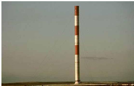
Figure 10: Manzanares SUT chimney
