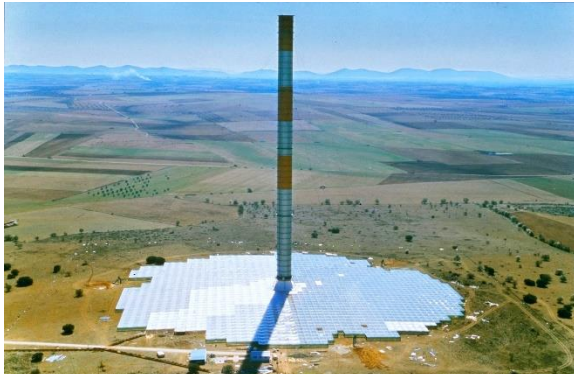
Figure 7: Manzanares solar power plant
