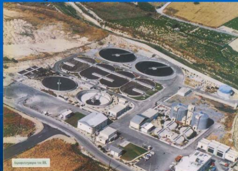
Biogas plant in Heraklion-Crete
